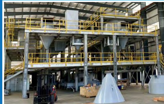
March 2024 – April 2025 Structural Steel Continues; Placing Milling & Shaping Equipment & Dust Collection
